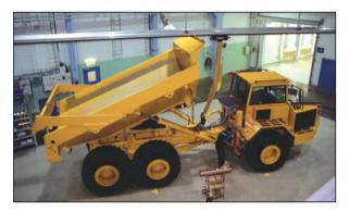
The STP can be mounted with the rail running parallel with the vehicle, which allows you to have full exhaust extraction from entrance door to exit door. This protects your workshop and its occupants from exhaust when operating vehicles. It can also be mounted along service bays for attaching to vehicles that are in stationary workstations.
